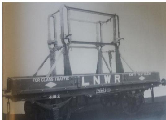
Initially glass was packed into wooden cases with the glass sheets standing on edge with the crates loaded onto ordinary open wagons and chained or roped down and sheeted over. As larger sheets became available specialist wagons were required and the LNWR addressed this by producing 6 different types between 1877 and 1909.
