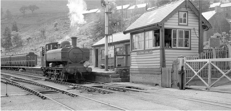
footplate. At that time, the coaches were still gas lit as the speed of the train was insufficient for a carriage dynamo to charge the lighting batteries.
