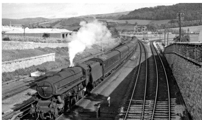
One of the distinctive final pair of Black 5's approaches Llandudno Junction station on the four track mainline with a Manchester-Llandudno express. The 27 mile single track Conwy valley branch to Blaenau, Ffestiniog curves away to the right.
